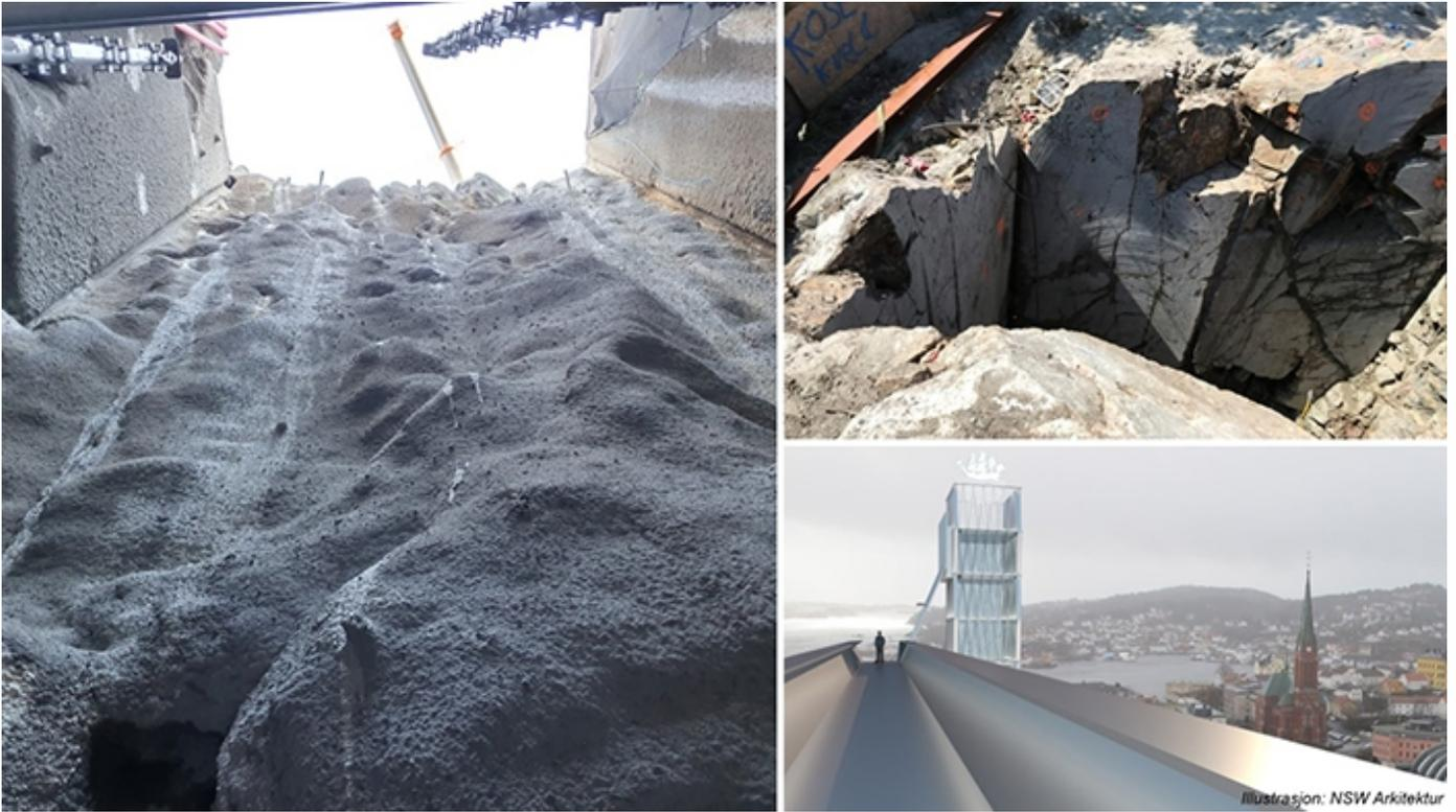
*Blasted and supported shaft (left). Top of blasted shaft (top right). Architect illustration of the footbridge with Arendal city in the background (bottom right).*
