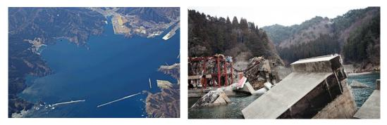
*Figure 11: Damage of the worlds' deepest breakwater in Kamaishi, left before damage, right, after damage (Source: <u>www.nytimes.com, http://community.</u> <i>guinessworldsrecords.com).*
