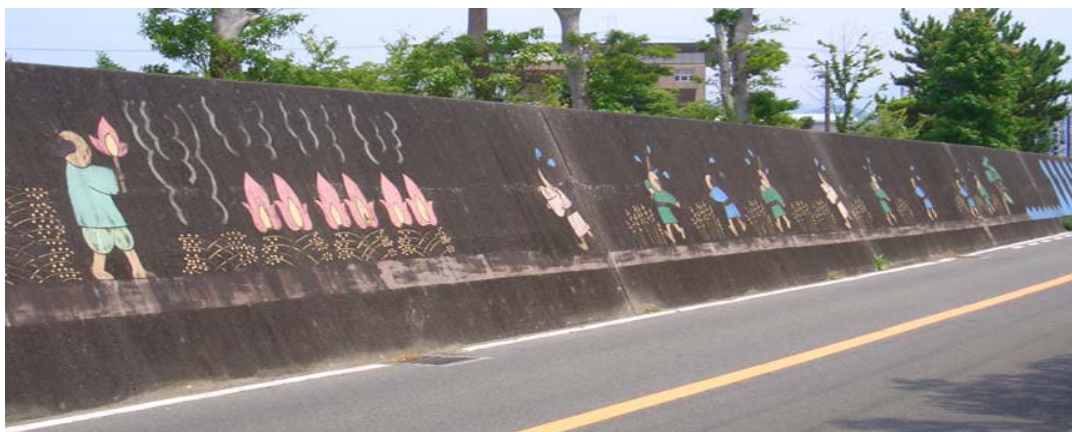
Fig. 2.1 600 m long and 5 m high dike in Hiro, Japan. The paintings remind of the 1854 tsunami which led to the building of the dike. Hiro was hit by another tsunami in 1946, but the almost 100 years old dike protected the community behind (modified from Ohta et al. 2005).
