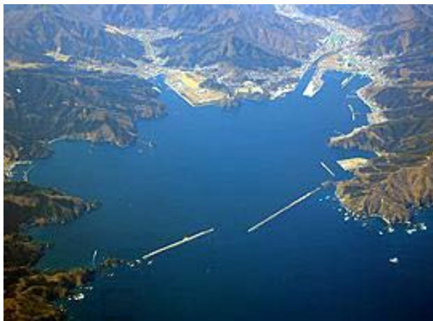
Fig. 2.6 Breakwaters at the entrance to Kamaishi Bay. (Source: PIANC Report N° 122, 2014)
