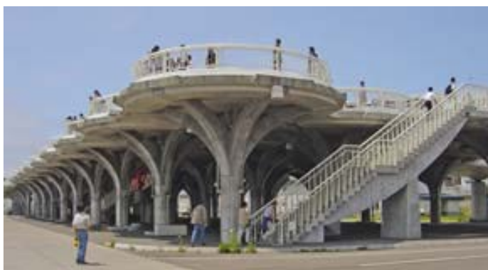
Fig. 3.7 Elevated platform used on Okushiri Island (Source: Scheer et al., Handbook of Tsunami Evacuation Planning, 2011. Retrieved from: http://ioc3.unesco.org/itic/printer.php?id=20 )
