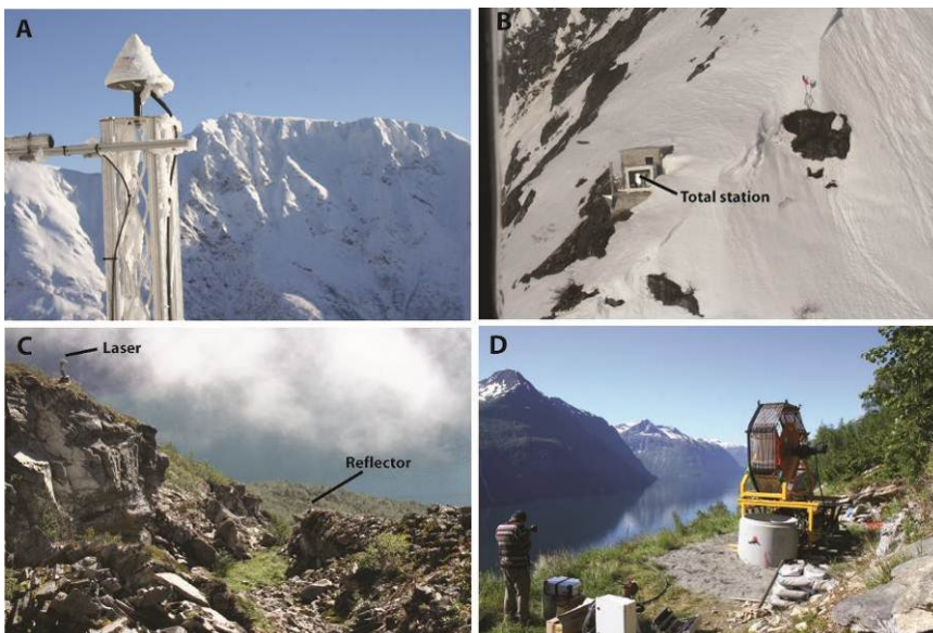
Figure 4.1-8. Selected monitoring systems at Åknes. A) GPS antenna B) Total station C) Single laser at the deep upper fracture D) Borehole DMS instrumentation.
