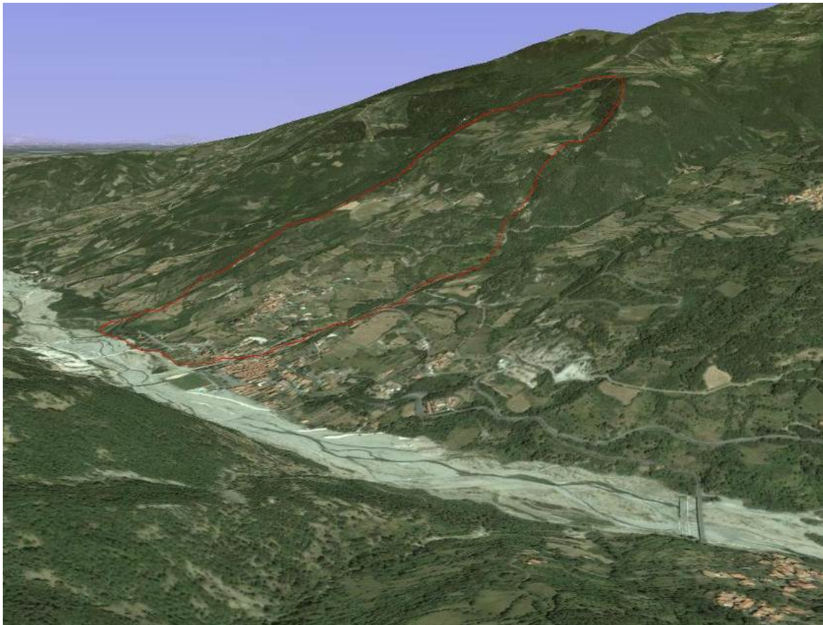
Figure 4.6-1. Casella landslide area.
