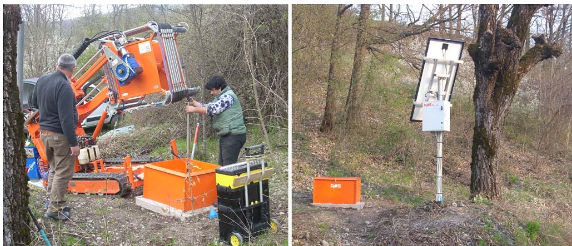
Figure 4.6-3. DMS system during and after installation.
