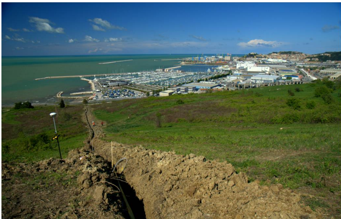
Figure 4.3-5. Installation trench of the monitoring profile.
