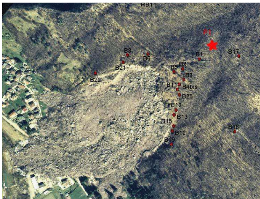
Figure 4.5–3. Aerial view of the Bindo-Cortanova rockslide, showing the main failure occurring in December 2002 and the location of optical targets.
