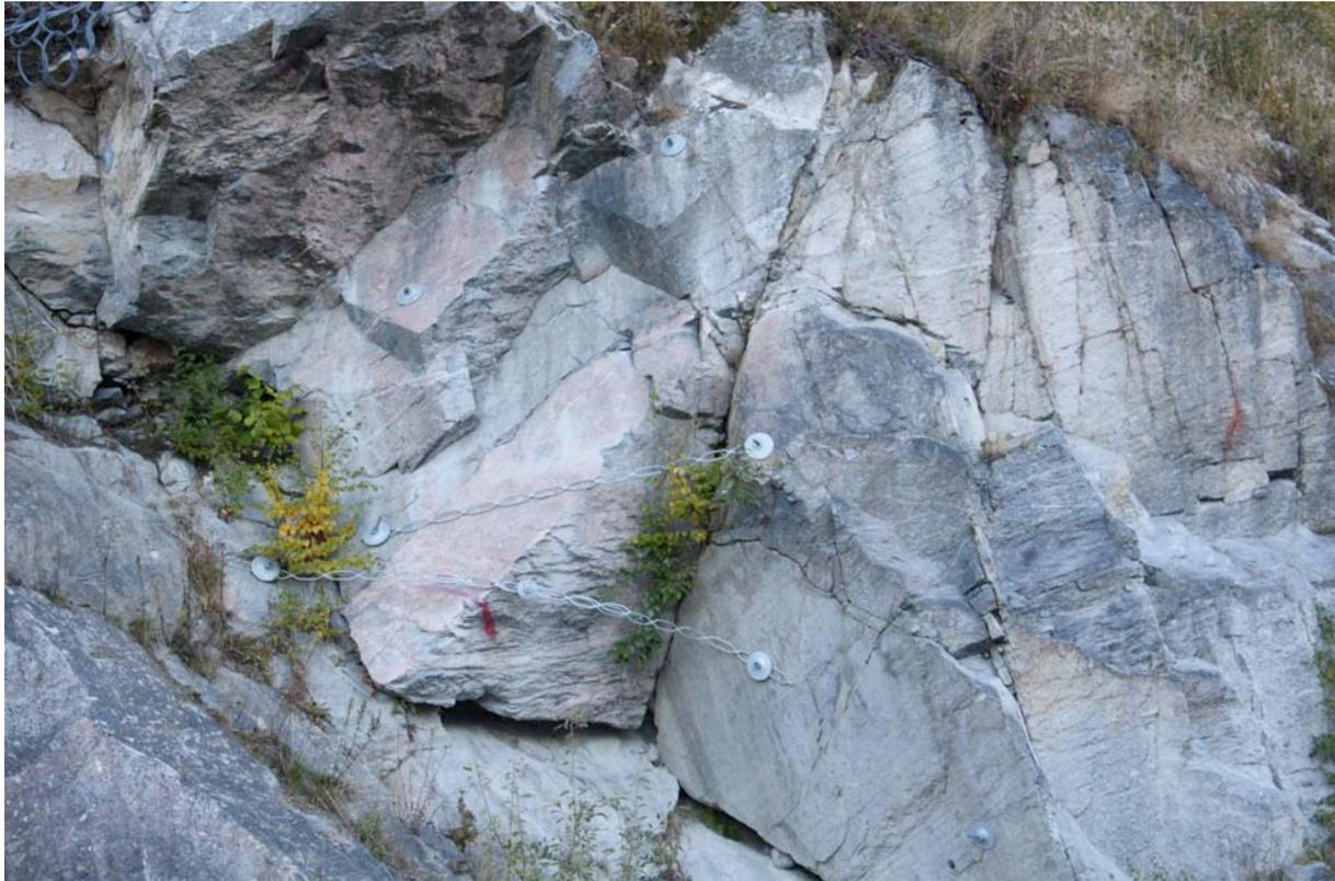
**Figure 118: example of an outcrop affected by an important fracturing; some anchors have been installed to stabilize the unstable blocks.**
