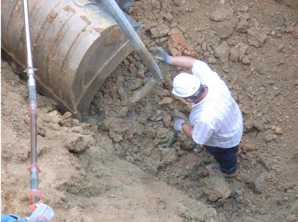
**Figure 80: DMS column removal (13th July 2009), and displacement check after excavation**
