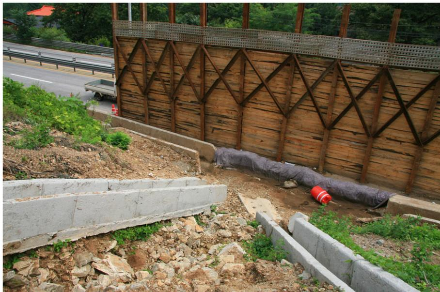
**Figure 4.5.25** Debris flow site from July 2009 at the Seoul to Chuncheon National Road 46 in the Republic of Korea. The barrier was erected after the event to protect the road from the effects of further flows while the concrete drainage channels were badly damaged during the event.
