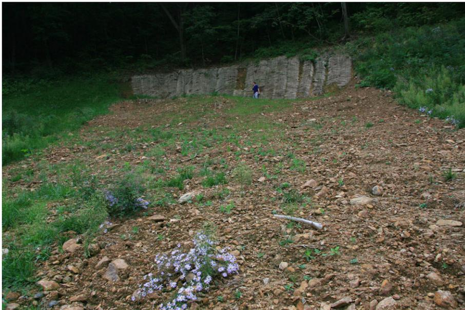
*Figure 4.5.28 Source area for a debris flow site from July 2009 above tunnel portals on the Seoul to Chuncheon National Highway in the Republic of Korea.*
