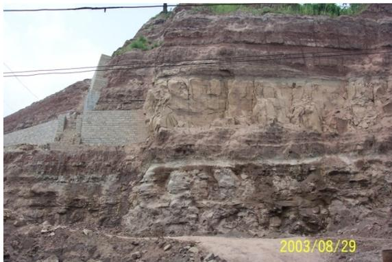
Figure.5 Soft interlayer of mudstone with rich montmorillonite
