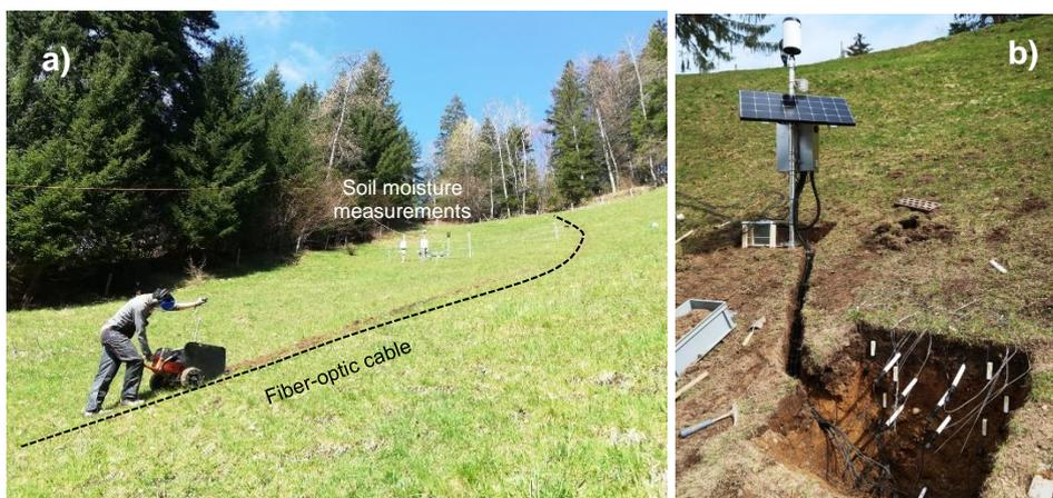
Fig. 2 a) Monitoring site Wasen i.E. with the installation of a fiber-optic cable for Distr. Acoust. Sens. (DAS) measurements; b) Set-up of the soil moisture measurements at Trub.
