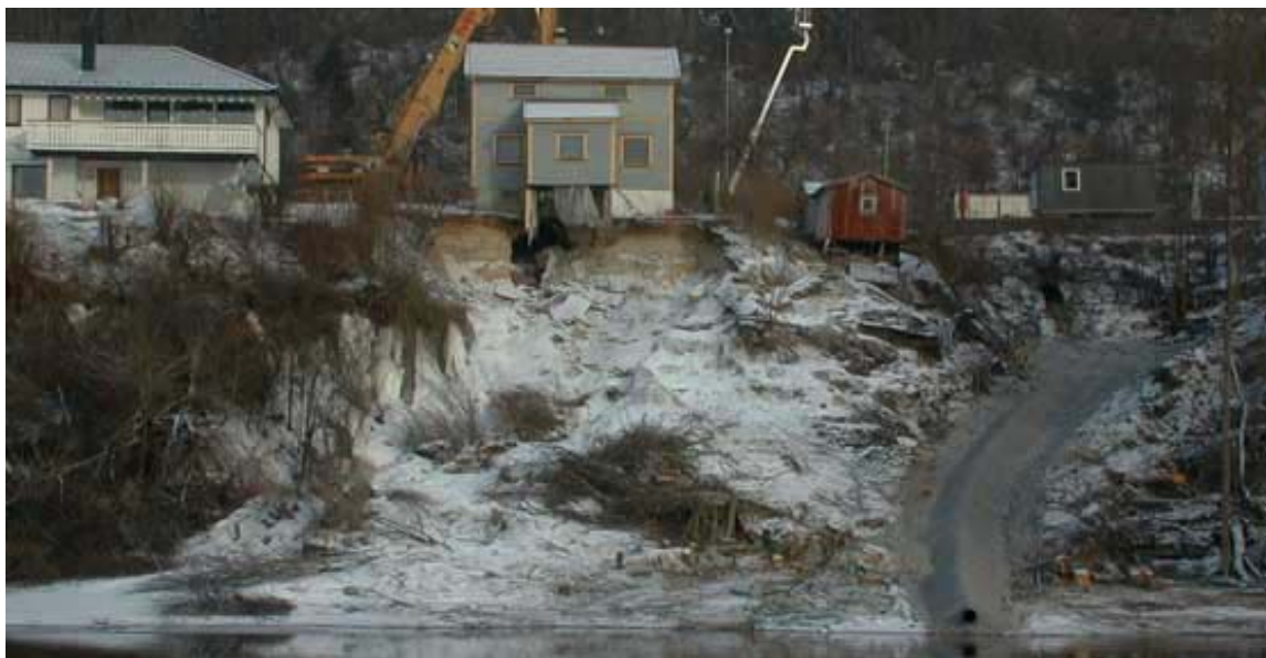
Figure 2 Clay landslide by the Skiens river. Foto: Skien municipality.
