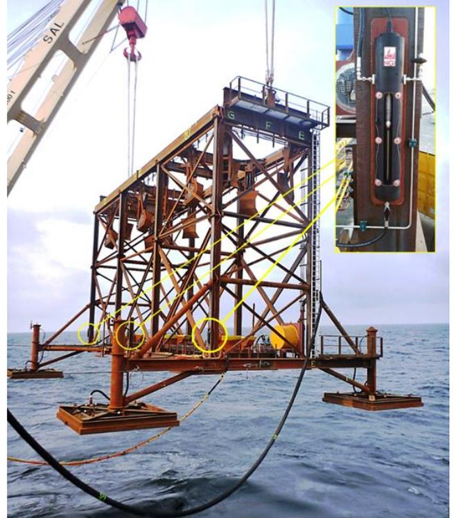
**Subsea self-levelling piling template with hose level system**
