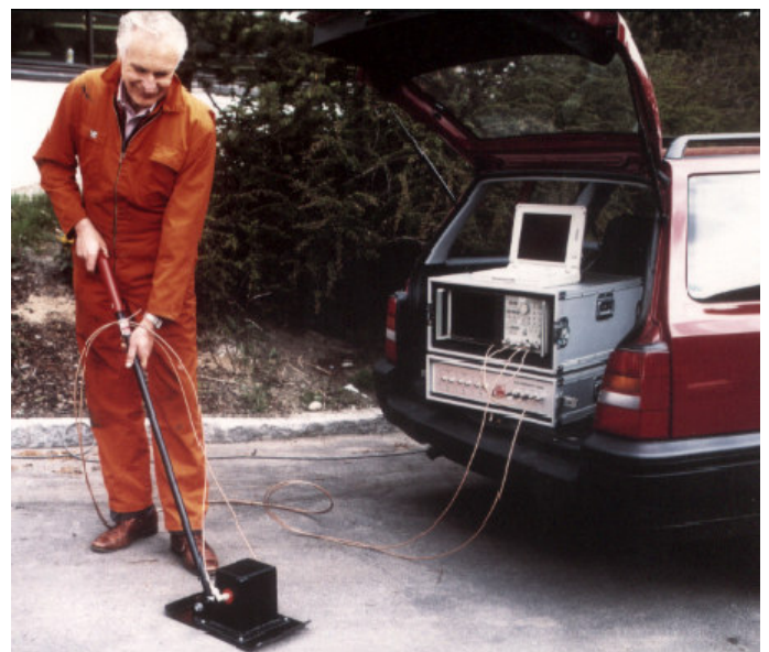
Figure 1. Pavement mapping using stepped frequency radar.
